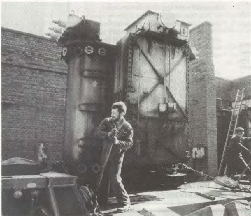
The first of the heavyweight transformers being winched on to the low-loader after having the oil coolers removed
