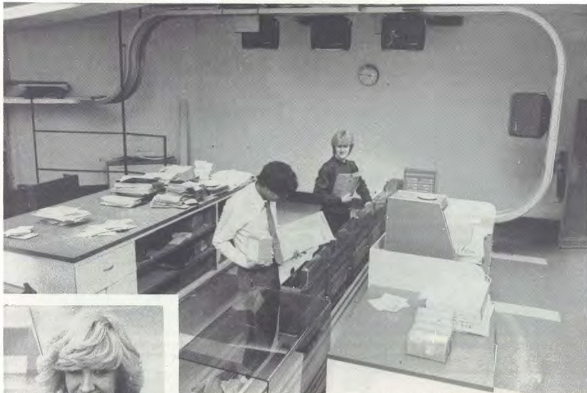
Above, Ray Morgan and Debbie Jones unload the 'Telelift' cars at the Mailing room terminal. On the twin track looping away in the background more cars wait their turn to come in to be emptied. Inset left, Karen Hunt loads a car to send on the 1/4 mile track to one of the five other terminals. Cars arrive at the fourth floor registry, above centre, and are unloaded by Caroline Buckley and Helen Gocher. Whilst on the second floor, top right, Jean Cannon and Carol Parry load a car for the mailing room.
